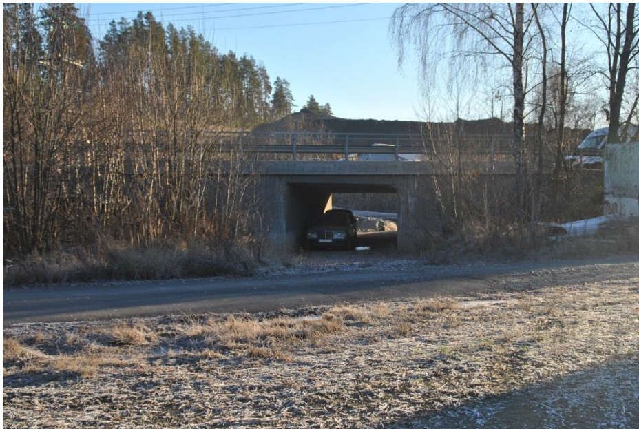
Figure 4.10: Underpass at southern branch of Lamyra. Picture taken 05.12.2018.
