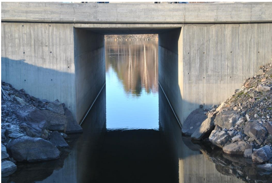
Figure 4.12: Box culvert at Juveren. Viewing direction to Storelva. Picture taken 05.12.2018
