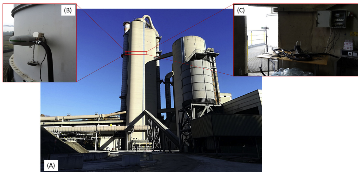
Fig. 2. Field test point in the cement plant, (A) grey clinker rotary kiln with its 5-stage cyclone pre-heating tower and the gas emission stack in Colacem S.p.A. cement plant located in Gubbio (PG), Italy, (B) Sampling point of the flue gas from the emission stack, (C) Permeation test rig located in the preheating tower.
