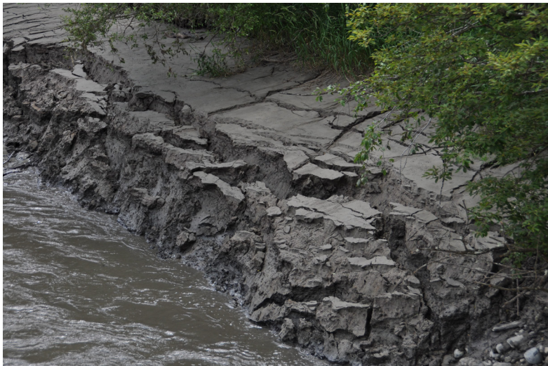
Fig. 1. Bank failure during flushing of the Bodendorf reservoir.
