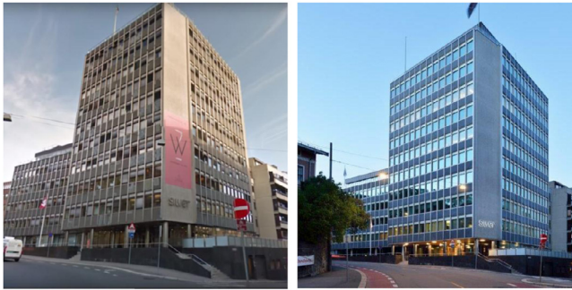
Fig. 8. The Wergelandsveien 7 building before (left) and after renovation (right).
