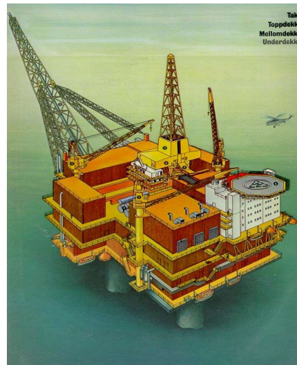
Figure 3. Large North Sea production platform with a petro-chemical process plant. (Courtesy Statoil)
