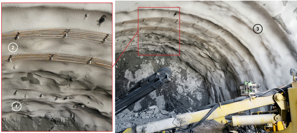
Fig. 1 Mounting of rebars for two RRS for permanent support (2). Further toward the face two (1) blast rounds are temporarily supported with spiling bolts held in place by steel straps and radial rock bolts. Finished RRS can be seen to the right (3).
