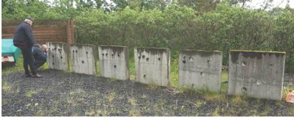
Fig. 1. Concrete walls at the Icelandic Building Research Institute (picture by Fournier, 2014).
