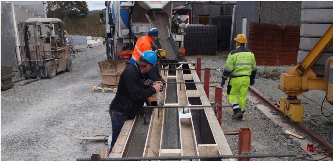
**Figure 2 Casting of wall elements from truck gutter**
