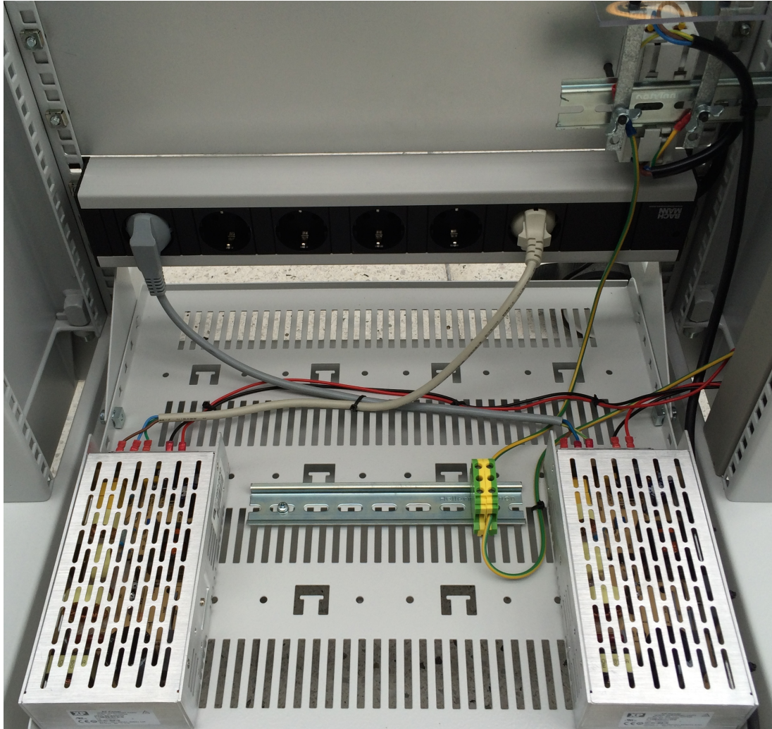
Figure 8.3.: Relay Power Supply
