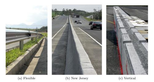
Figure 1.: Barriers used in the present study. (a) metallic, (b) and (c) concrete.
