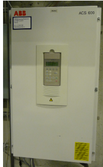
Figure 25: The ABB frequency converter used to emulate wind.
