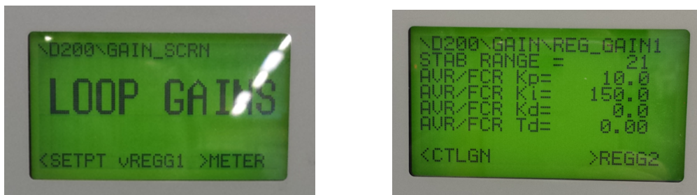
Figure 73: Generator Protection Unit: AVR settings
