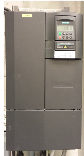
Figure 30: The frequency converter controlling the induction motor.
