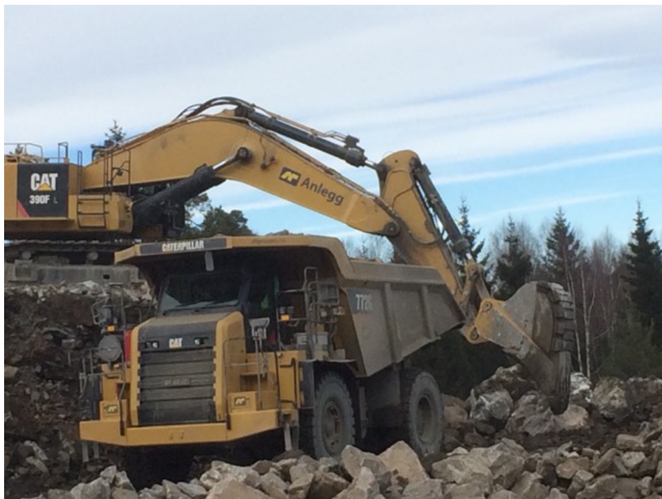
Figure 3.3: CAT 390F loading a dumptruck, Tvedestrand-Arendal forbindelsen - AF Gruppen AS
