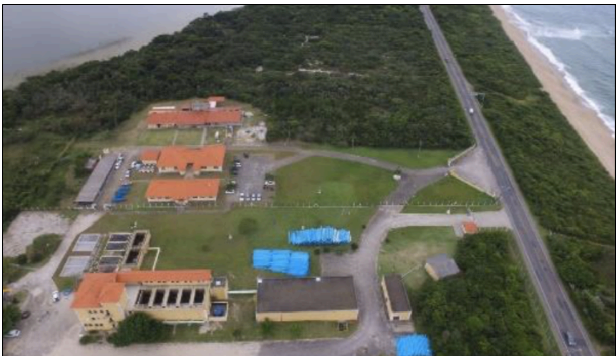
Figure 3: Location of the WTP at Lake Peri (Source: CASAN, 2016)
