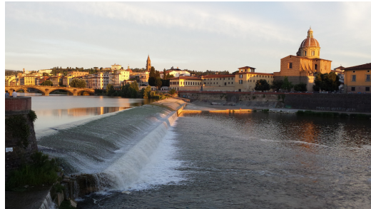
(e) Downstream Santa Rosa weir
