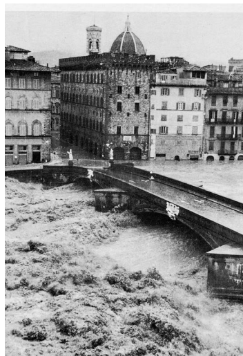
(c) Santa Trinita bridge
