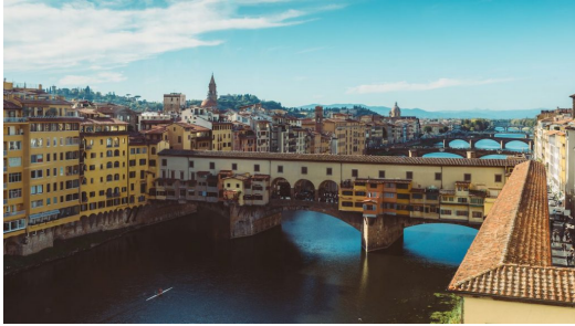
(a) Upstream Ponte Vecchio
