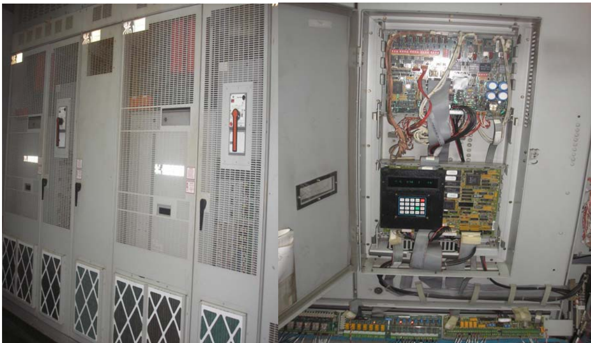
Photo 4.8: The static excitation system, EX2000, at Takoradi Thermal Power Station,
