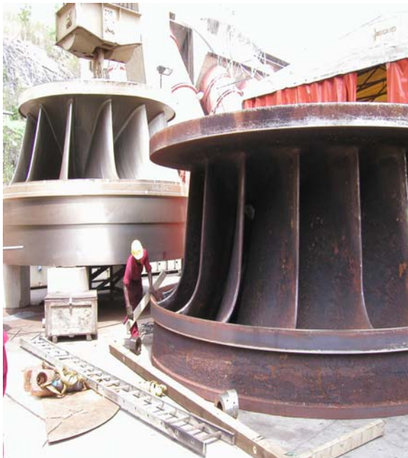
Photo 1.2: New stainless steel turbine used to replace the old turbine during retrofitting of Akosombo GS. The capacity of the plant was increased from 912MW to 1070MW
