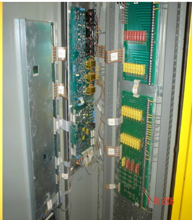
Photo 4.6: Master card of Akosombo exciter with PSS circuitry having dual input, speed and electrical power
