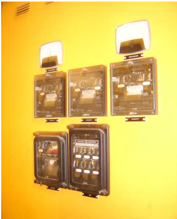
Photo 4.5: Silco 5 static excitation System from GE for Akosombo generating units equipped with PSS
