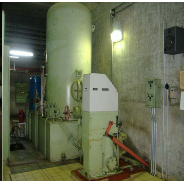
Photo 4.3 :Electro-hydraulic governor of Kpong GS manufactured by Asea.
