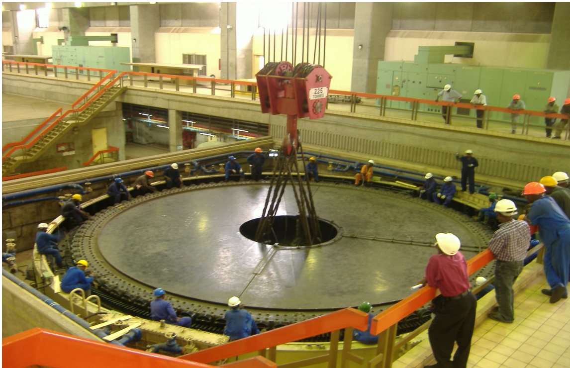
Photo1.5: Refurbishment of a 40MW unit at Kpong Hydro Generating Station. Removal of salient pole rotor
