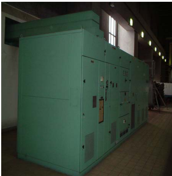
Photo 4.2: Static electronic exciter of Kpong Generating Station manufactured by Toshiba. This exciter is not equipped with PSS
