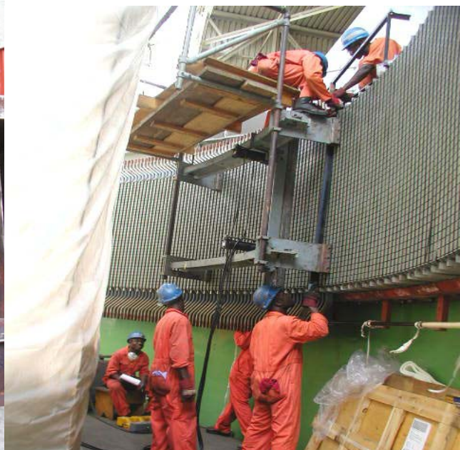
Photo 1.3: Rewinding of generators for increased capacity during retrofit of Akosombo GS
