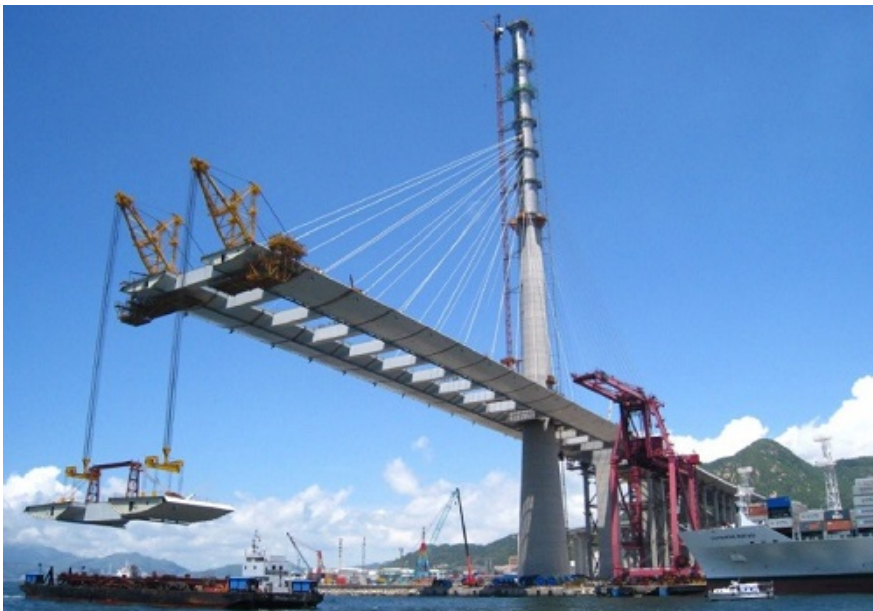
Figure 2.11: Building of Stonecutters Bridge (USA 2013) [2].
