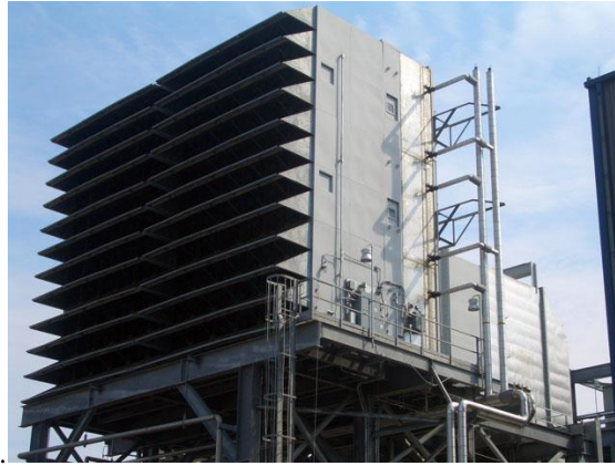
Figure 13: Inlet hoods on offshore gas turbine.
