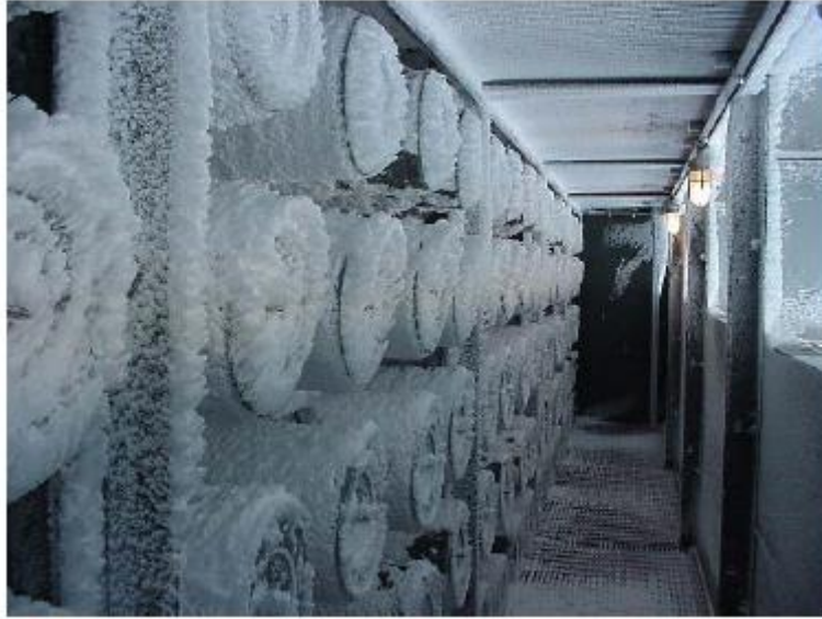
Figure 10: Picture of ice build-up in cartridge filters [16].
