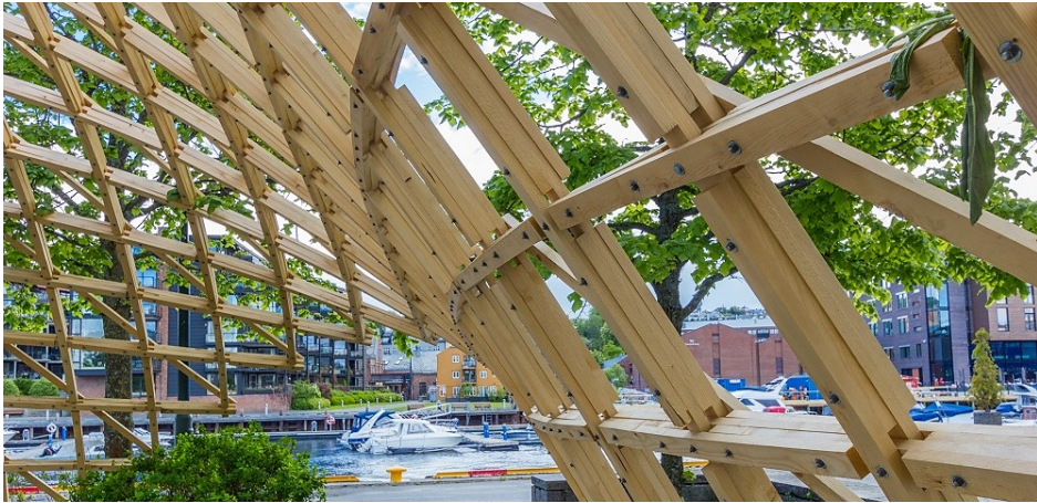
Figure 1.6: Kinematic Gridshell from Trondheim Pavilion, [8].
