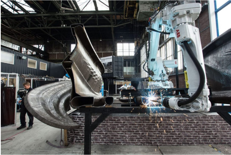
Figure 1.8: The MX3D team 3D-printing a steel bridge, [13].
