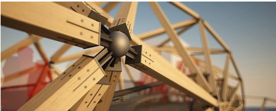
Figure 2.7: Ball joint used in Roppe Bridge project in Romania, [29].
