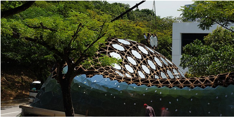
Figure 2.10: Overview of the SUTD Library Pavilion project, [32].
