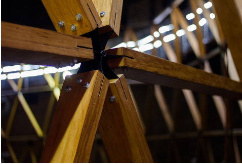
Figure 2.13: Detail from The Wooden Geodesic Dome in St. Petersburg, [10].
