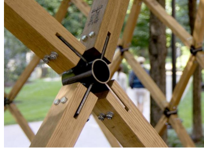
Figure 2.12: Lo-Fab Pavilion, connection detail, [33].
