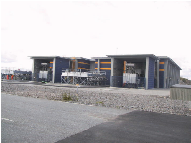
Figure 16: Kollsnes HVDC Light converter station (Source: ABB)
