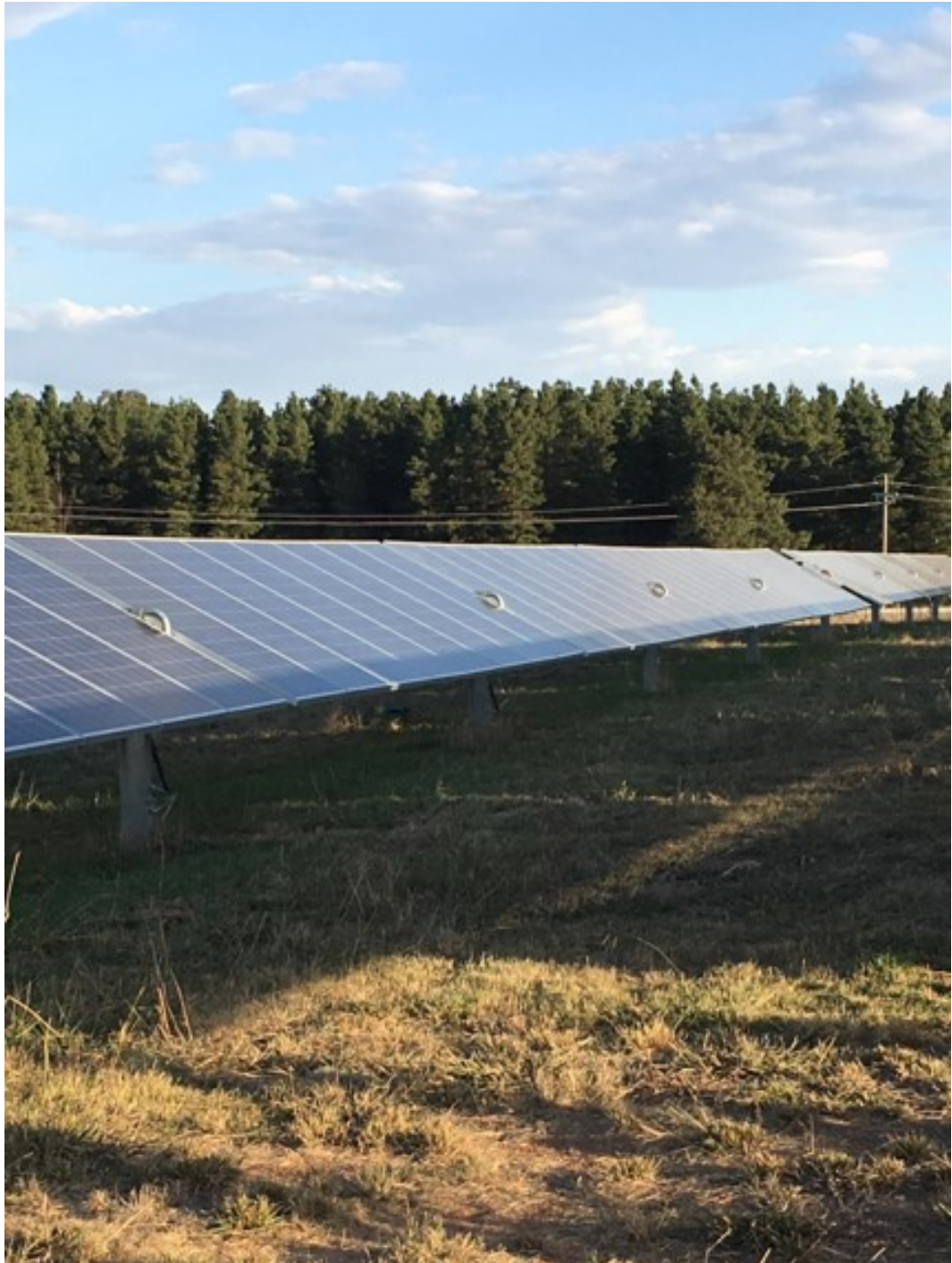
Fig. 2.3. Self shading of a SAT system [28]
