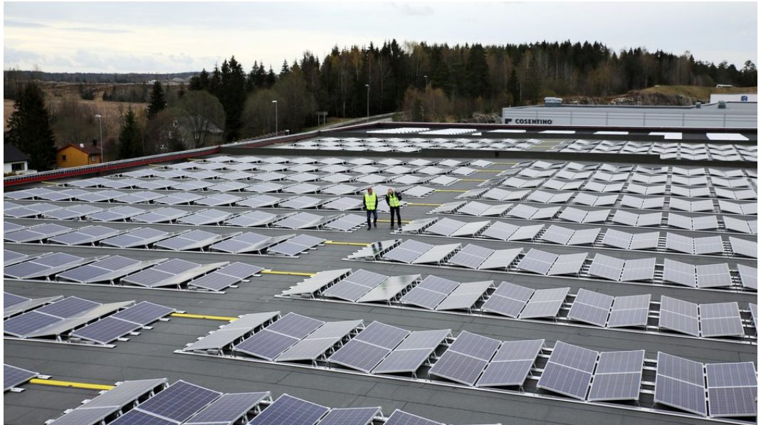
Fig. 6.35. Commercial PV installation in Norway with panels facing east/ west tilted 10^\circ [67]
