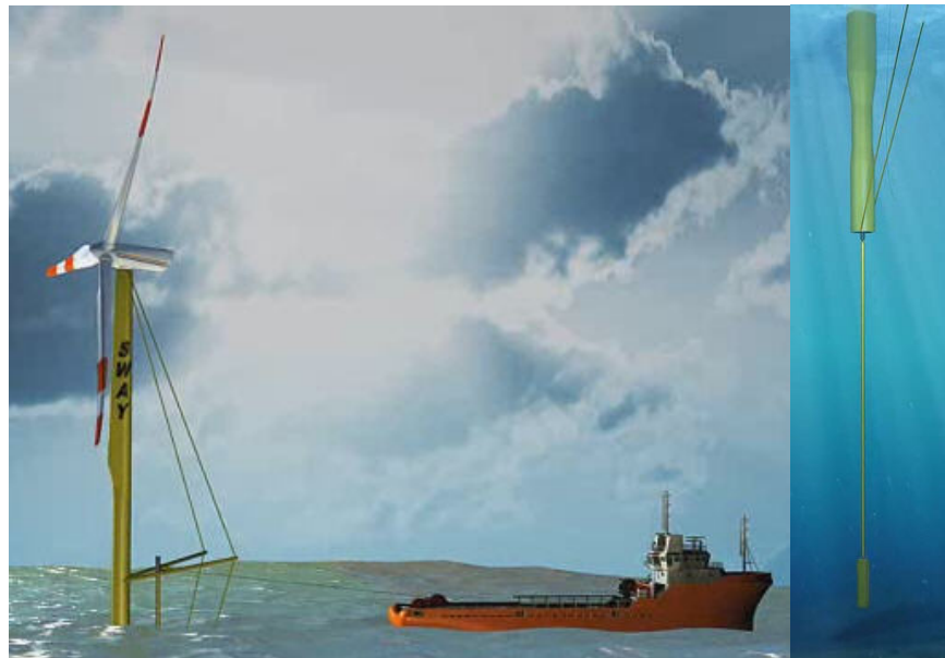
Figure 1-14: SWAY project, tow of a floating turbine (left) and view on the mooring tensed leg (right).
