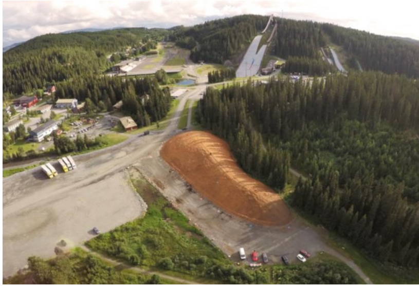
Figure 3.2: Snow storage covered with sawdust in Granåsen (Vagle, 2017)
