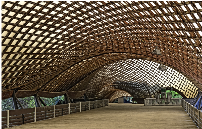
Figure 1.4: Inside the Multihalle in Mannheim. Shell structure with a double-layered lattice grid [9, Fig. 12.1]
