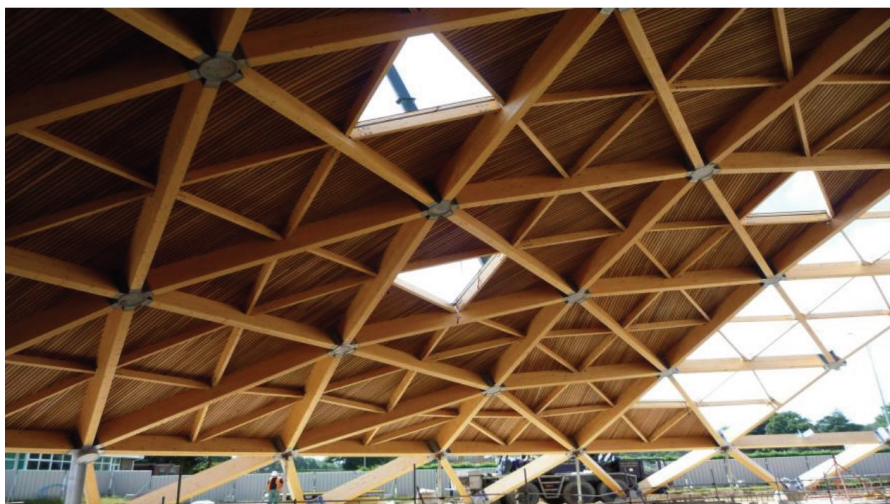
Figure 1.7: Reticulated shell roof of The Pods [14, Fig. 24]
