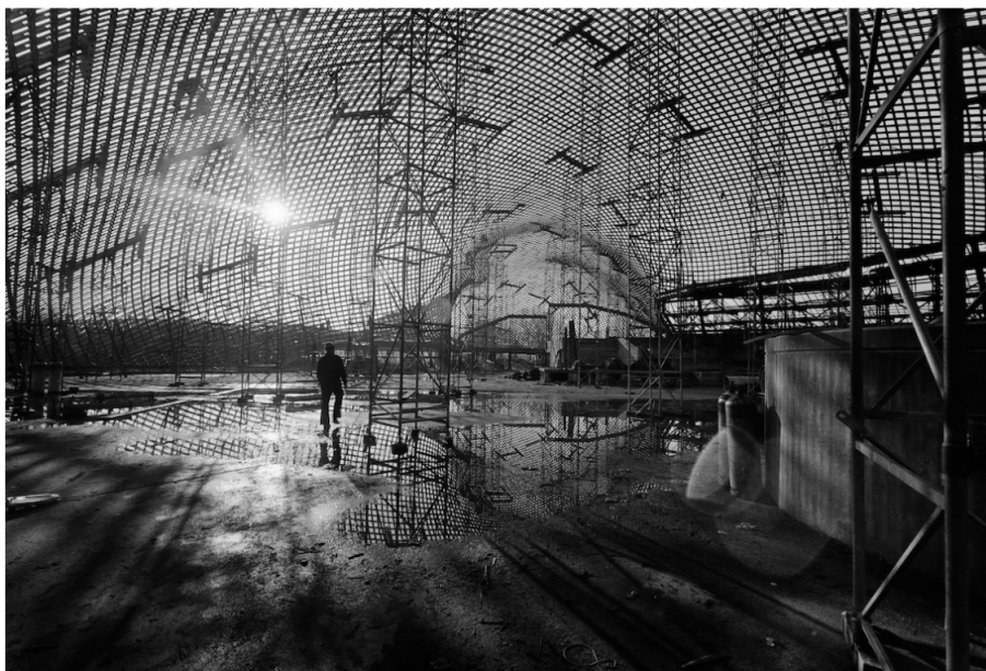
Figure 1.5: Interior shot of the erection of Multihalle in Mannheim [12]
