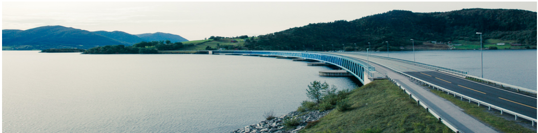
Figure 2.2: Bergsøysund Bridge, Møre and Romsdal, Norway (NTNU, 2017)
