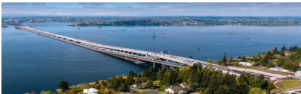
Figure 2.1: Evergreen Point Bridge, Washington State (Marshall, 2016)
