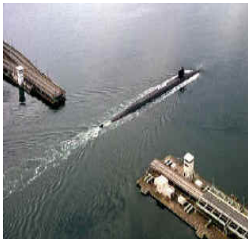
Figure 2.5: Drawspan on Evergreen Point floating bridge, Washington, USA (Jembatan, 2013)
