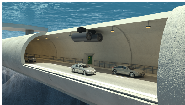
Figure 2.7: Inside view of the Submerged Floating Tube Bridge [NPRA and NVF, 2017].
