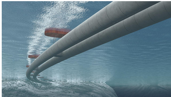
Figure 2.6: General underwater view of the Submerged Floating Tube Bridge with pontoons [NPRA and NVF, 2017].
