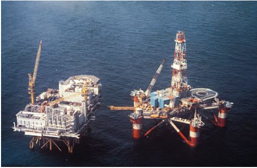
(a) Alexander Kielland platform before the accident
