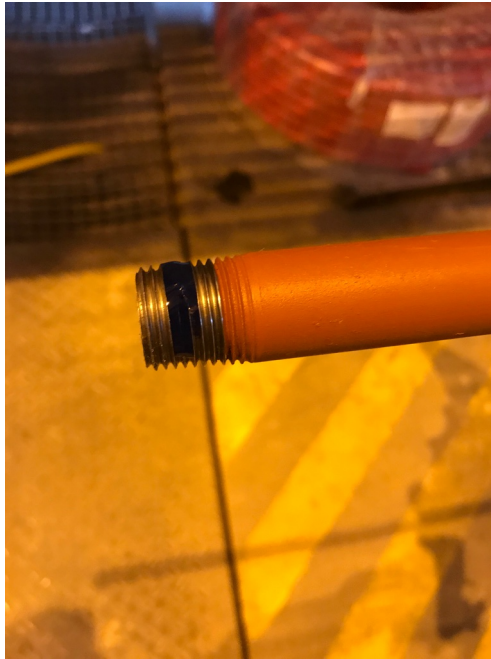
Figure E.15: Sealing adhesive applied to drillpipe
