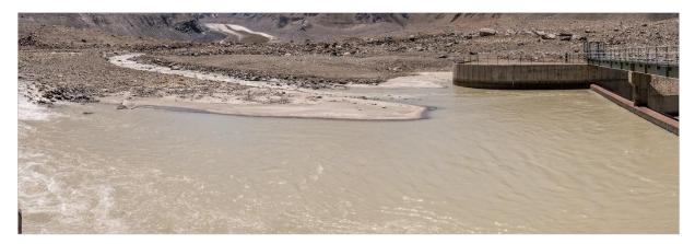
The regulation pond has a surface area of 1.9 ha and a total storage capacity of 115,000 m<sup>3</sup> (ARCADIS Geotécnica, 2010). Although its main aim is to allow hydropeaking operation, its dimensions allow it to also performs a de-sanding task of the flow coming from the intake.
