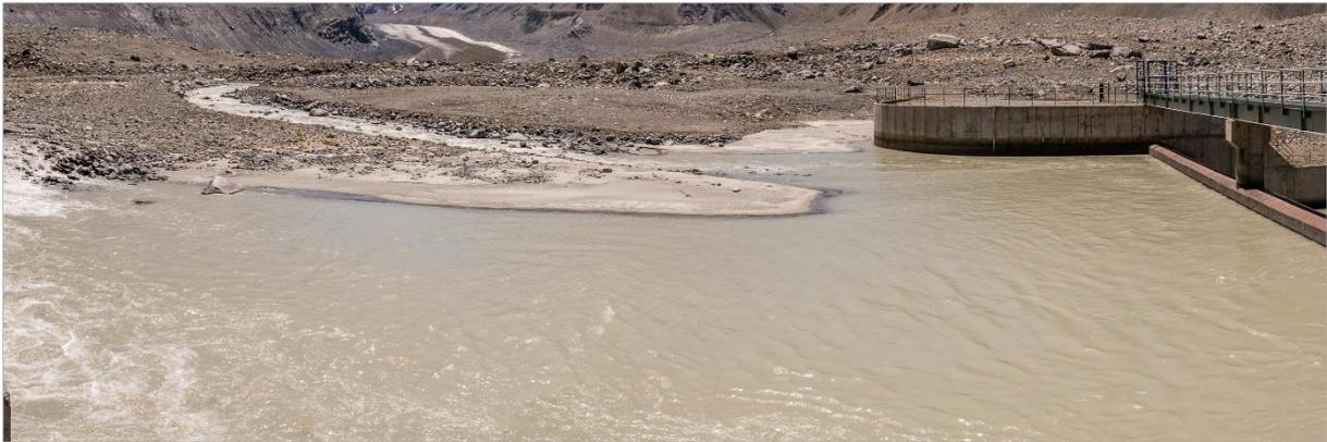
The regulation pond has a surface area of 1.9 ha and a total storage capacity of 115,000 m<sup>3</sup> (ARCADIS Geotécnica, 2010). Although its main aim is to allow hydropeaking operation, its dimensions allow it to also perform a de-sanding task of the flow coming from the intake.
