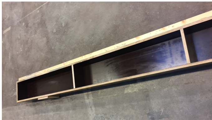
Figure 4.2: Beam formwork
