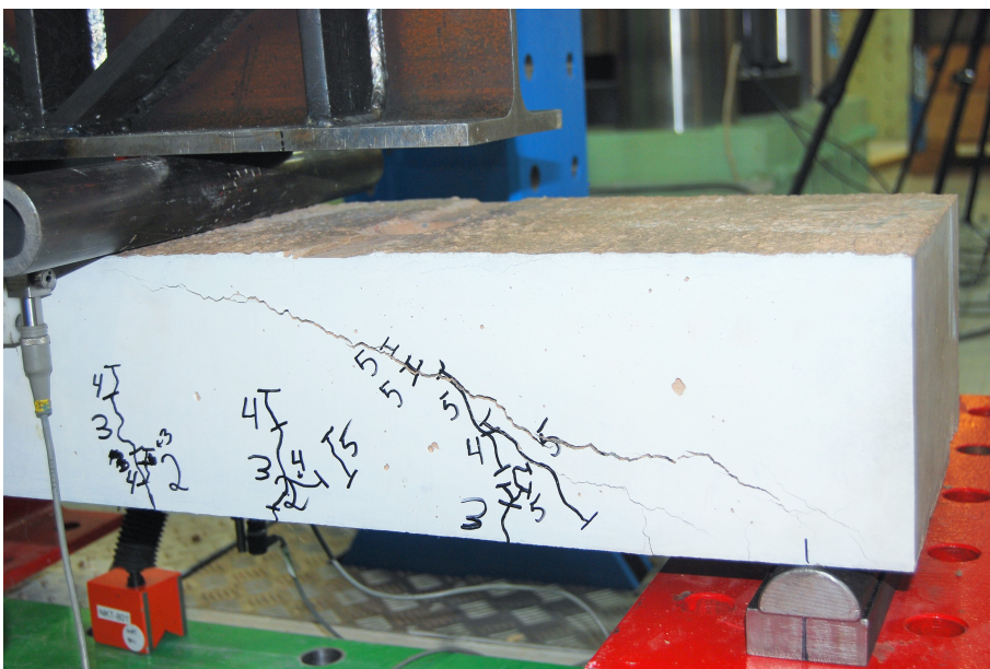
Figure 6.2: Shear failure of beam B2-2ø12-STEEL
