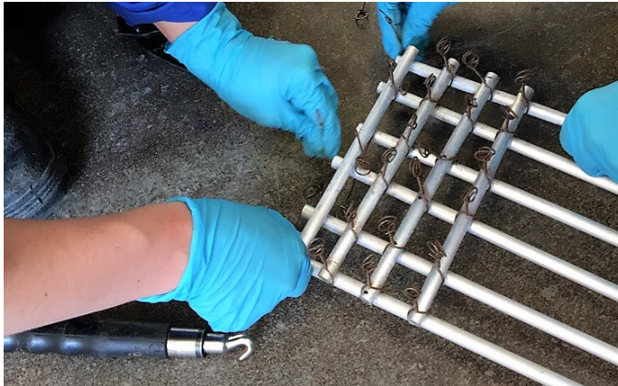
Figure 4.3: Binding of the aluminium reinforcement
