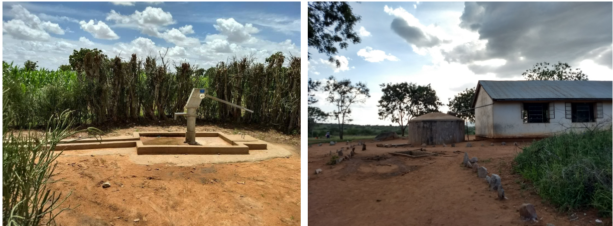
Figure 7-3: 1: India Mark II hand pump. 2: Rainwater harvesting tank in Munguli primary school.
