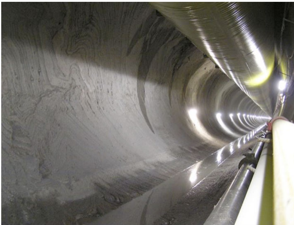
Figure 6.4: TBM excavation of the unlined headrace tunnel at Glendoe (Reynolds, 2017)
