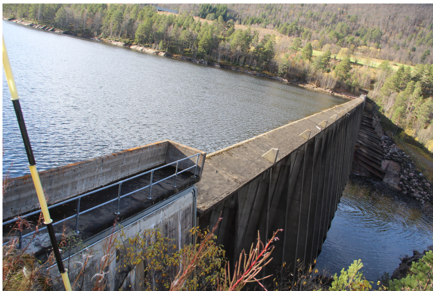
Figure 7.4: The Storfoss dam and reservoir at the intake of Brattset HPP
