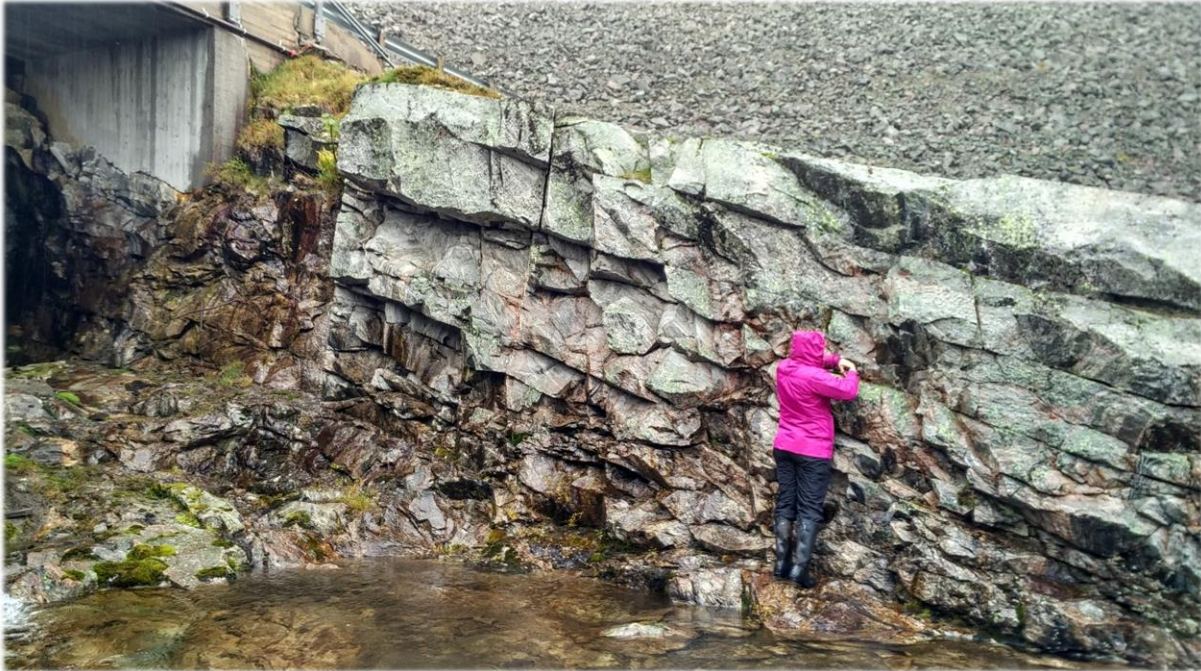
Figure 28 - Measuring joints close to the added tunnel and the dam of Roskreppfjorden. (Bibek Neupane)
