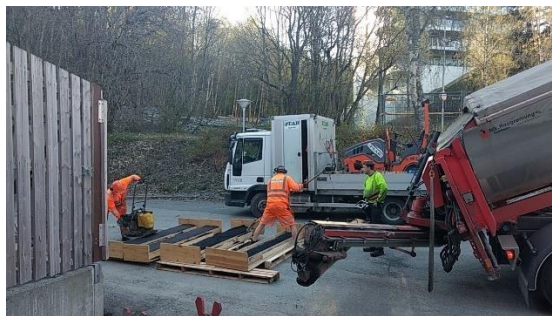
Figure 47 - Layering of asphalt done by Peap Asphalt Norge AS.
