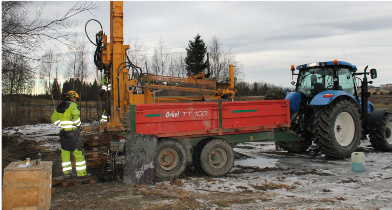
Figure 2.4: The drill rig was elevated above ground level using a trailer.
