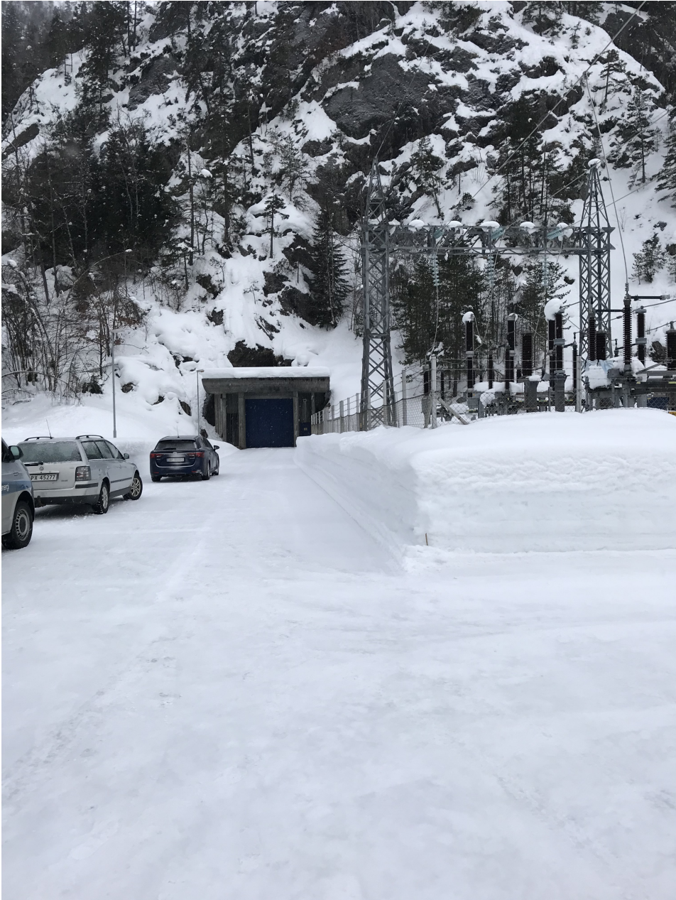
Figure 1.3: Entrance to Smeland power plant
