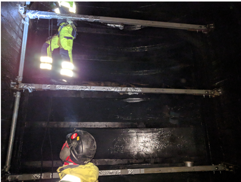
Figure 3.5: Frame used in outlet, 3 individual beams
