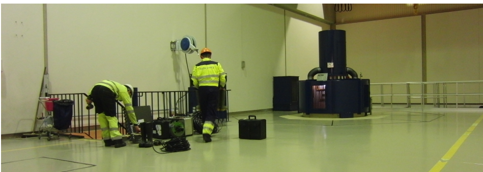
Figure 3.1: Unloading the equipment at Smeland power plant
