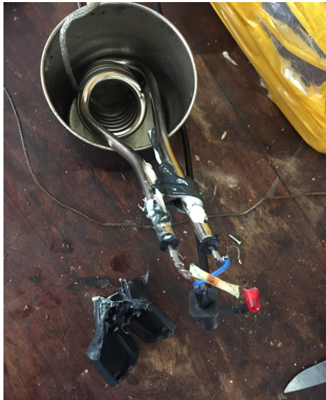
Figure 4.19: Melted heating element
