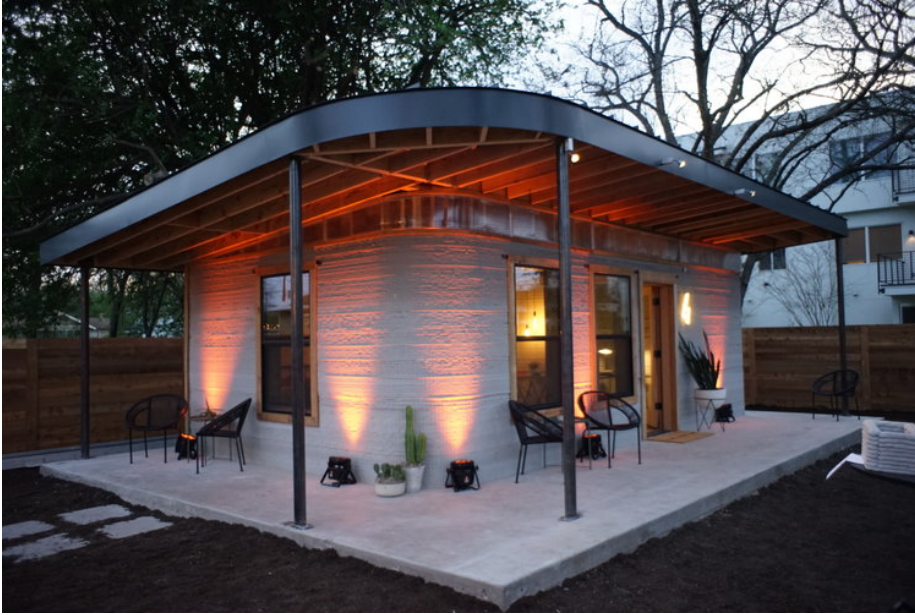
Figure 2.2: New Story + ICON: 3D printed house. Image courtesy of New Story + ICON: 3D printed houses (2018)
