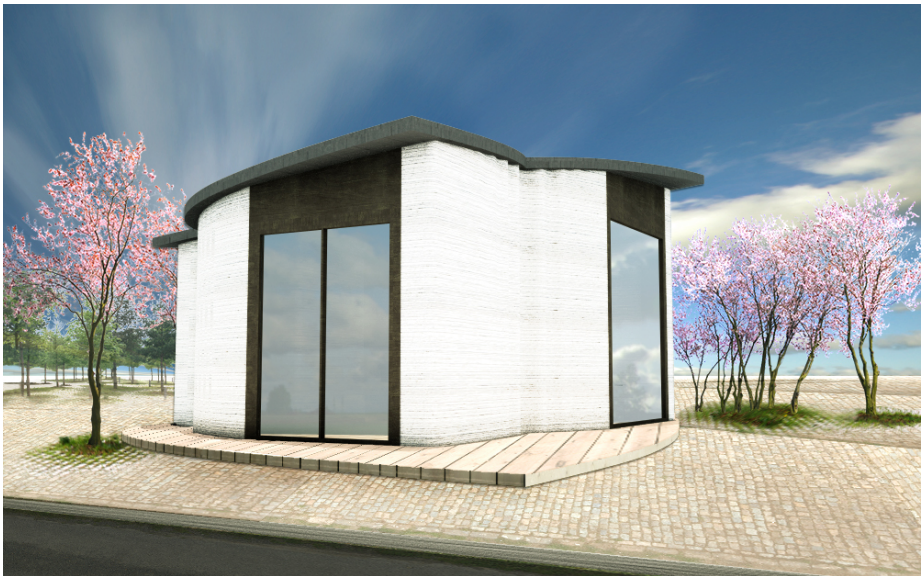
Figure 2.1: The BOD. Image courtesy of The construction of Europe's first 3D printed building has begun (2017)
