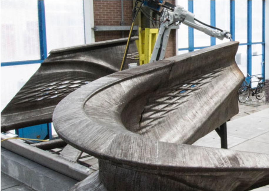
Figure 2.4: MX3D Bridge Project - Robot on bridge. Image courtesy of MX3D (2018).
