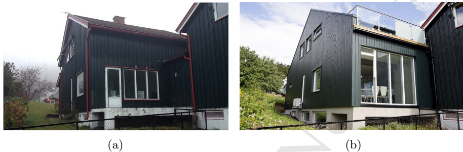
Figure 2: Pictures of the single-family house analyzed: (a) before and (b) after the renovation works. Reprint with permission [SINTEF Byggforsk]; Copyright 2018, http://seopp.net/forside/ .
