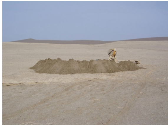
Photo 2 Top of a vertical shaft of a karez
