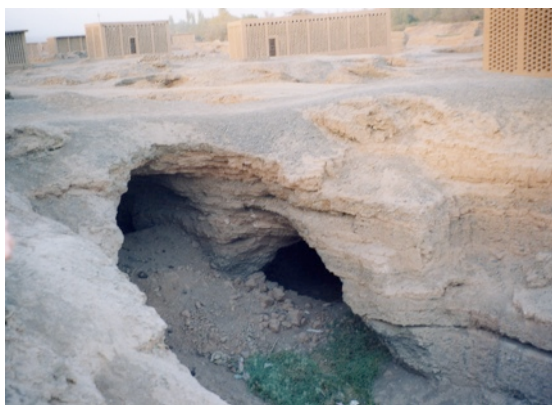
Photo 1 Collapsed karez with two water supply tunnels
