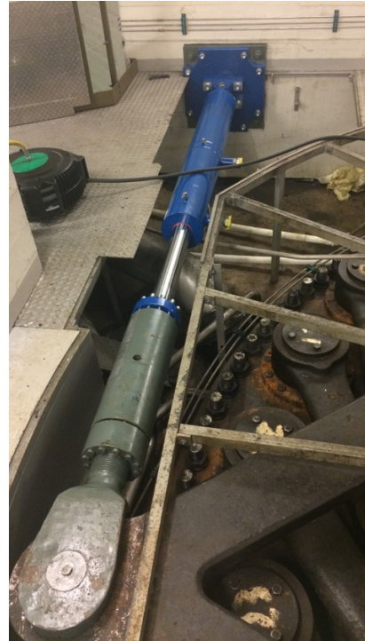
Figure 1.4: Hydraulic actuator for guide vane control. The actuator is mounted to a ring that controls the guide vane opening. Courtesy of Hymatek Controls
