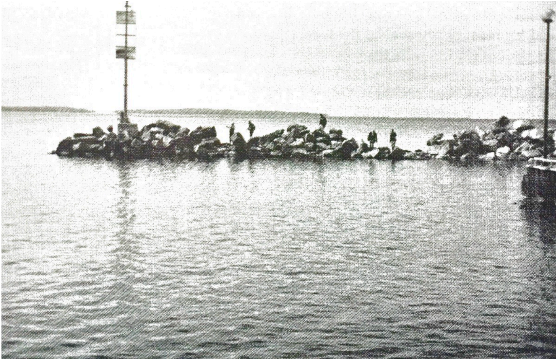
Figure 2-7 Sections of this breakwater have been ‘bulldozed’ during an ice event one winter [19].
