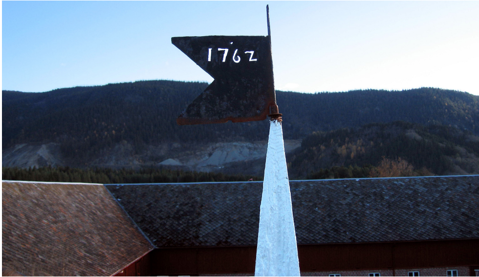
Figure 3.15: 1762, is written as an inscription on top of one of the farm buildings. This gives clear indications that the building is over 250 years old.
