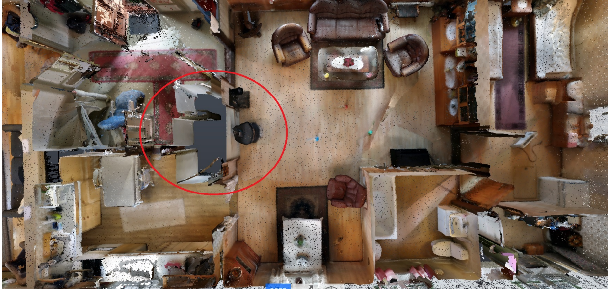
Figure 4.9: The first floor, on the southern part of the building displayed from above. When looking at the scan from such a view, it is possible to see the size of various objects: For example, parts of the chimney is placed in the middle of the red circle in this figure.
