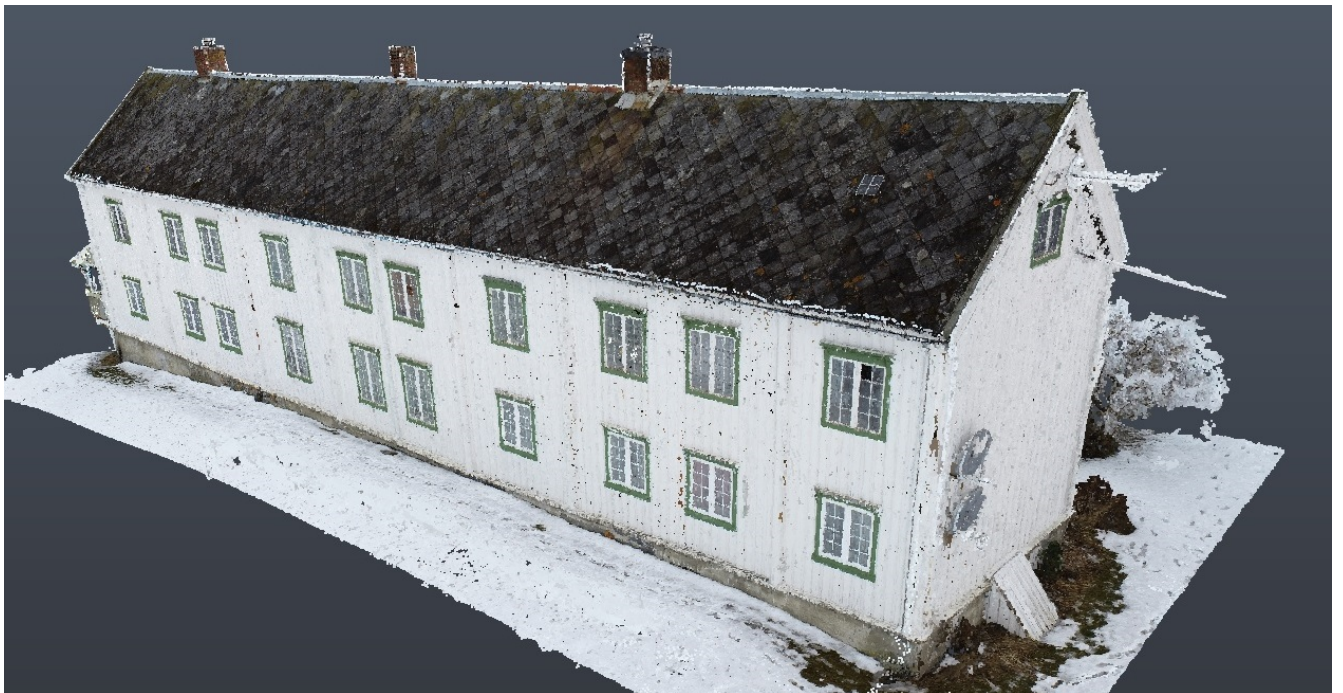
Figure 4.3: The Farmhouse viewed from South-West.
