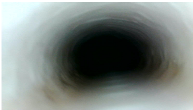
Figure 7.48: Picture taken 15cm inside copper pipe, outlet side
