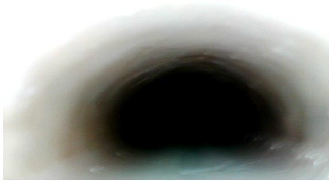
Figure 7.11: Picture taken 15cm inside copper pipe, inlet side
