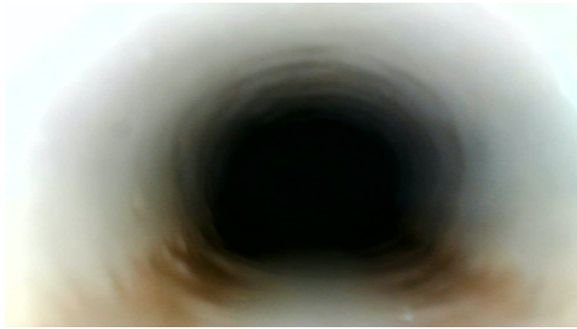
Figure 7.23: Picture taken 15cm inside copper pipe, inlet side
