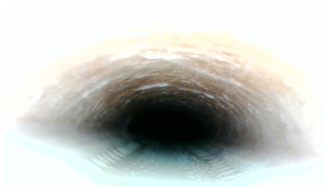
Figure 7.39: Picture taken 15cm inside copper pipe, outlet side
