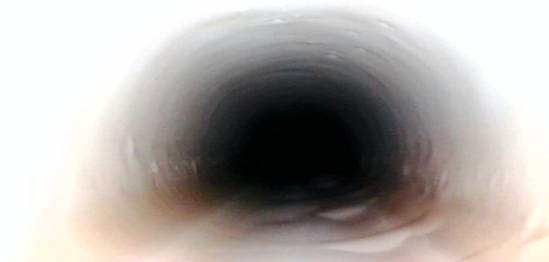
Figure 7.9: Picture taken 15cm inside copper pipe, outlet side
