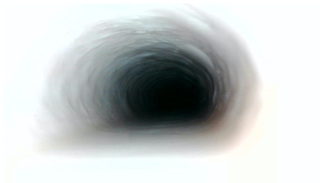
Figure 7.18: Picture taken 15cm inside copper pipe, outlet side
