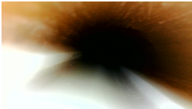
Figure 7.32: Picture taken 15cm inside copper pipe, inlet side
