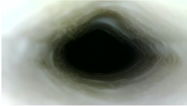
Figure 7.51: Picture taken 15cm inside copper pipe, outlet side
