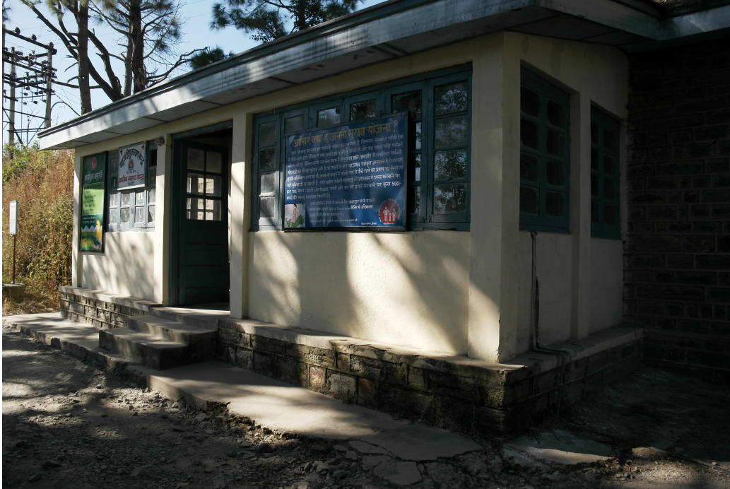
Figure 4.3: A sub centre in Shimla, Himachal Pradesh
