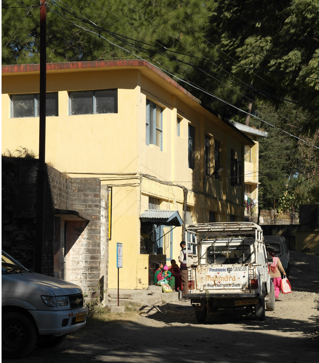
Figure 4.4: A primary health centre in Shimla, Himachal Pradesh
