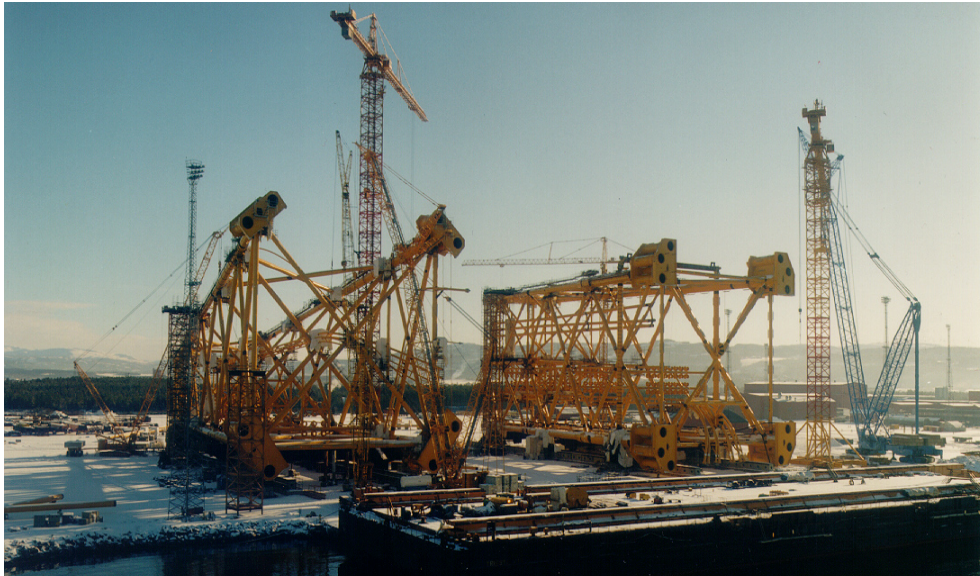
Figure 8.1: Assembled steel jackets at Aker Verdal
