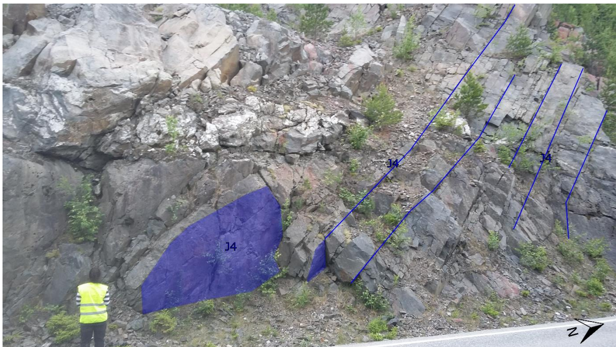
Figure 42: J4 observed at location D1 dipping into the slope.
