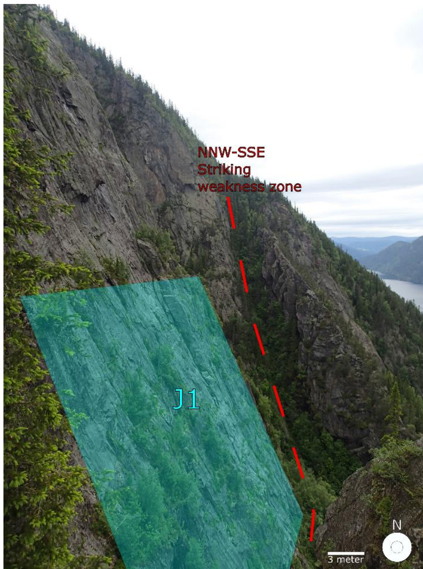
Figure 40: J1 and the NNW - SSE striking weakness zone oriented along the release surface of the Prestura rock slope failure, seen towards north.
