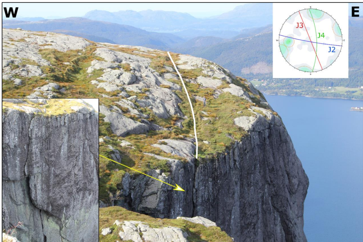
Figure 4.19: Main picture shows the depression intersecting the east flank with an open crack. Inserted figures show the fracture continuing down the cliff face, and that the depression follows a significant structure in the eastern domain, J4.
