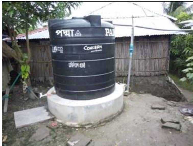
Figure 4:1 Rain water harvesting tank (sample 1)
