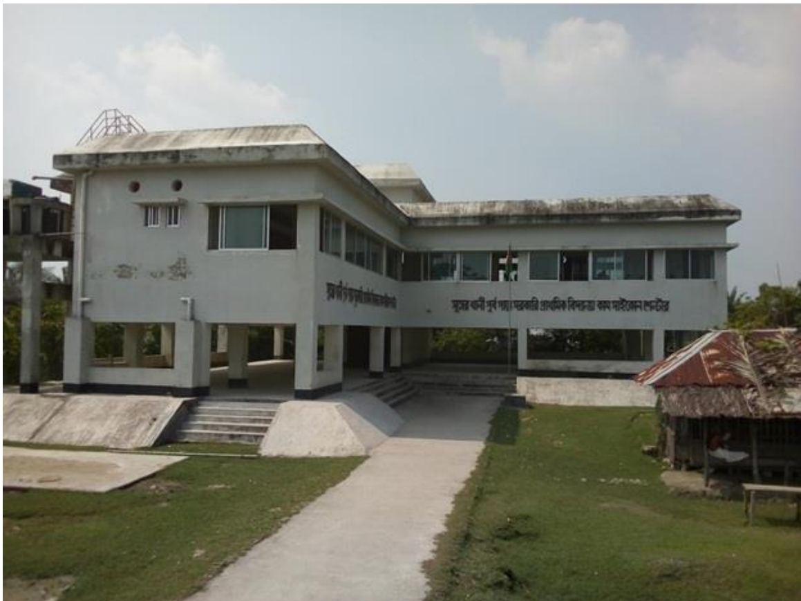
Figure 3:10 Cyclone shelter of Sutarkhali Union
