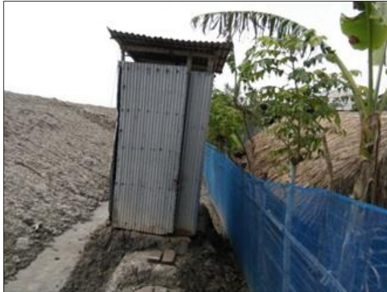
Figure 4:8 Image of pit latrine with slab and water seal
