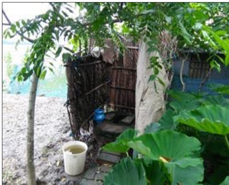
Figure 4:7 Image of latrine with open pit
