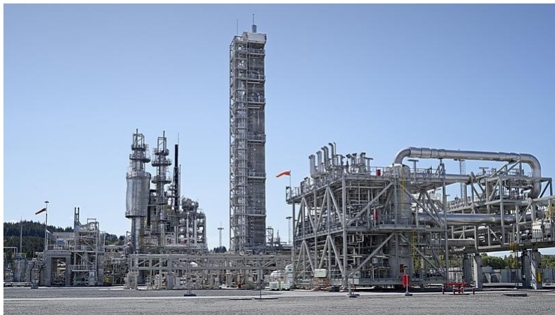
FIGURE 3.7: Amine pilot plant at Technology Centre Mongstad. Image obtained from ( The Third MEA Campaign at the CO 2 Technology Centre Mongstad ). To the right the direct contact coolers. In the centre the absorber column (64-m-height) and to the left the two stripper columns.
