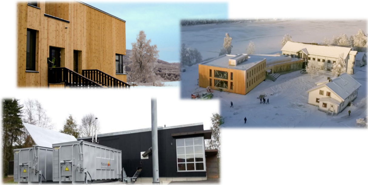
Figure 22 ZEB pilot building – Campus Evenstad, educational bldg. and offices (photos: Statsbygg).
