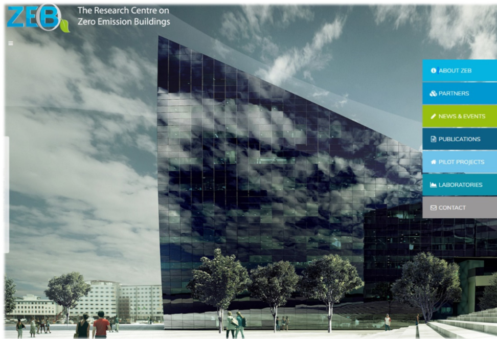
Figure 15 Powerhouse Brattøra, Trondheim – a plus energy office building under construction, January, 2018. (ZEB 2017)
